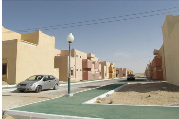
SOCIAL HOUSING PROGRAM ALGERIA EPC
