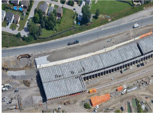
WINDSOR-ESSEX PARKWAY PROJECT CANADA EPC
