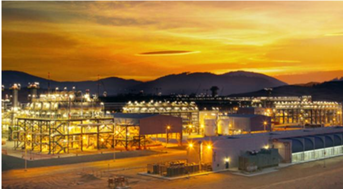
AL HOSH GAS DEVELOPMENT Oil & Gas Processing EPC
