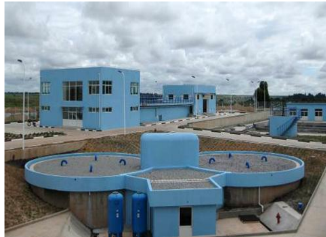
KUITO WATER SUPPLY WORKS ANGOLA
